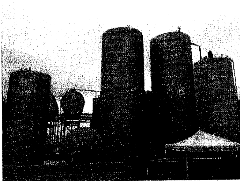
Above - DBWT - Triazine Tank assembly in Texas.
