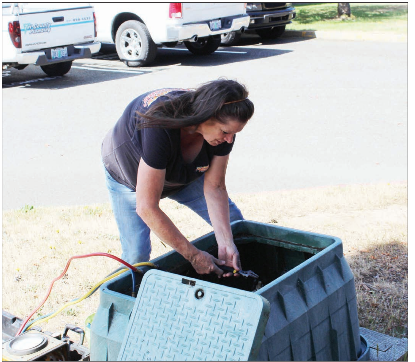
Elaine Plummer with Tri County Plumbing conducts a backflow test at the North Bend Municipal Pool. The backflow test is a mandatory requirement before the pool can reopen. Photo by David Rupkalvis/The World
