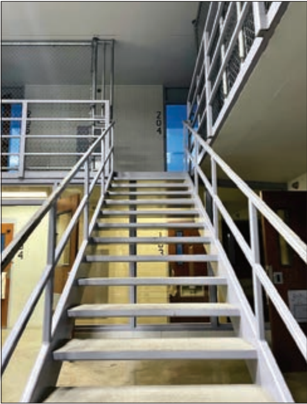
Photo courtesy of the Coos County Sheriff's Office The stairs are in one of the portions of the Cell Block 2A at the Coos County Jail, which opened Saturday, April 27, leading to an upper tier of rooms. The fencing on the upper tier is in place to prevent people from jumping or throwing items from above, Sheriff Gabriel "Gabe" Fabrizio said.
