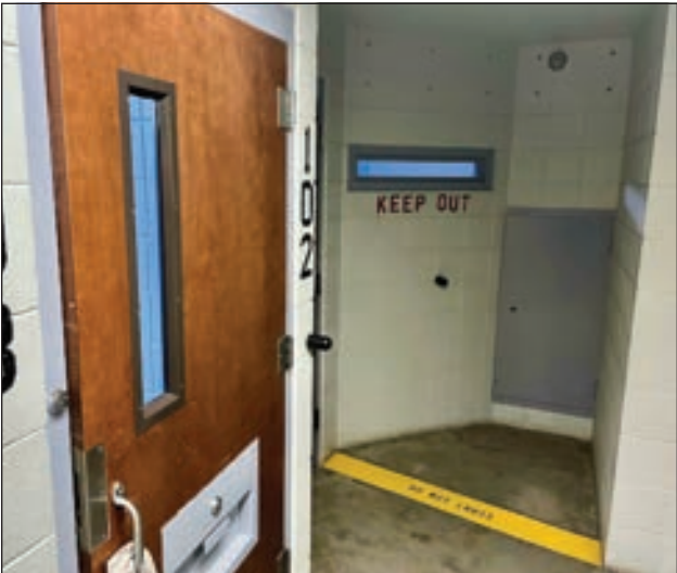
Photo courtesy of the Coos County Sheriff's Office This corner room at the Coos County Jail can be used for an Adult in custody who needs to be isolated.
