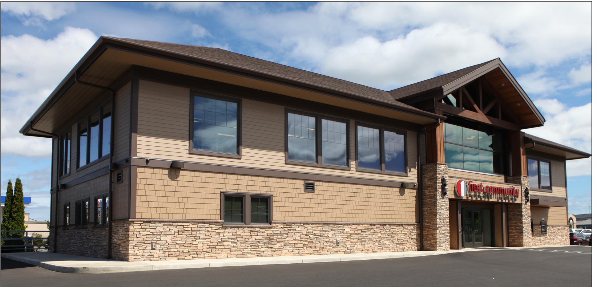
A remodel of the First Community Credit Union branch in Coos Bay recently completed.
