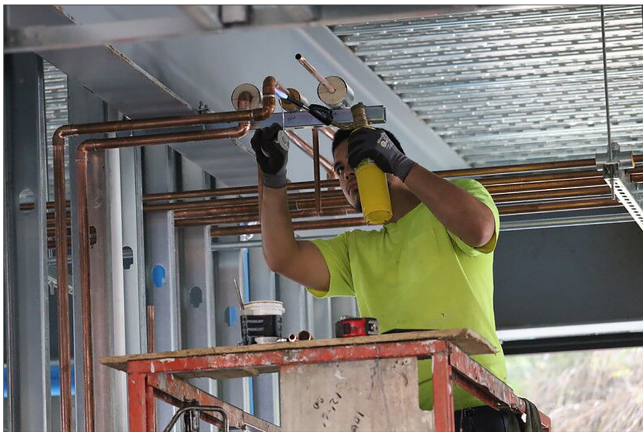
A worker does some piping work in the new Health & Science Building.
