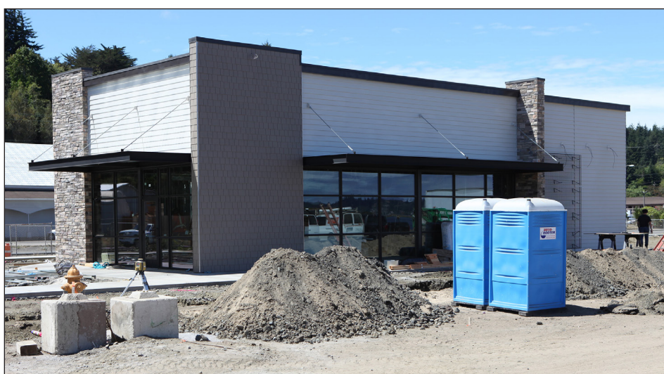
A Starbucks coffee shop with a drive-through window is one of the first buildings to be constructed in the Coos Bay Village complex.
