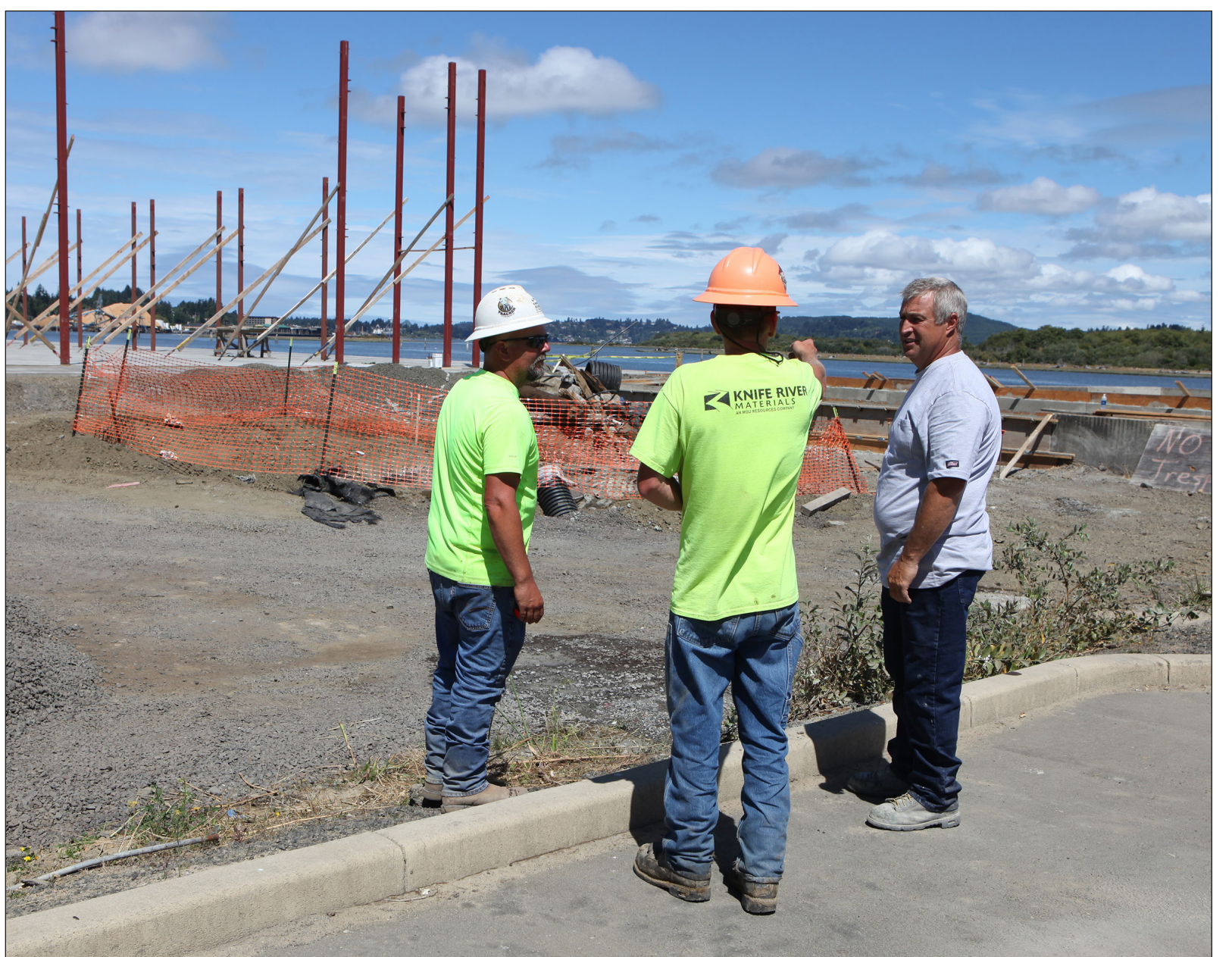
Daniel Graham, right, who is partnering with Greg Drobot on the Coos Bay Village project, speaks on the job site with contractors from Knife River Corp. who were working on placing underground utilities on Aug. 20. Drobot and Graham built Face Rock Creamery in Bandon and continue to own and manage the business.
