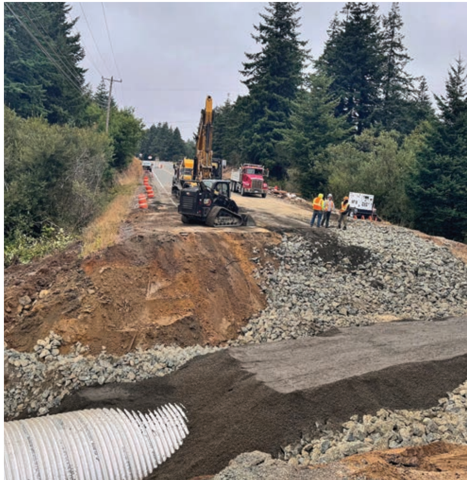
Re-opened: U.S. 101 was closed nearly 40 hours for the replacement of a failing culvert at Bearhead Mountain Lane, about six miles south of Bandon, Oregon. Prime Contractor Farline Bridge, Inc. and the Oregon Department of Transportation reopened the highway at 12:20 p.m. on Sunday, Sept. 21, 2025, about eight hours ahead of schedule. Photos courtesy of ODOT
