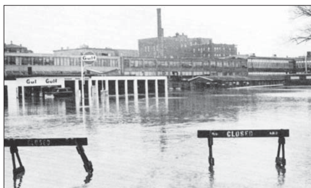
Flooding temporarily closed the L.G. Balfour Co., plant in Attleboro in 1968.
