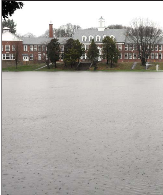
The field in front of Willett School in Attleboro flooded during historic rainfall and flooding in March 2010.
