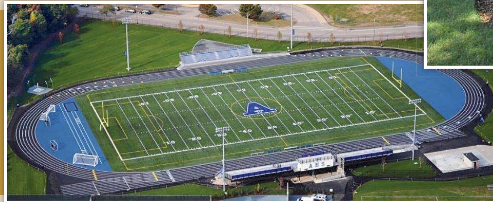
Attleboro High School Stadium ▲
