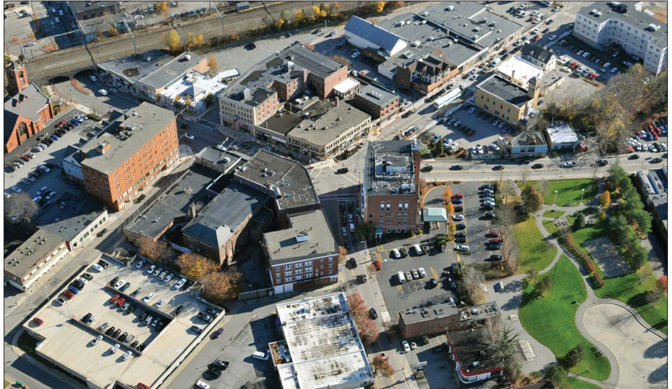
Downtown Attleboro with the Balfour Riverwalk in the bottom right.
