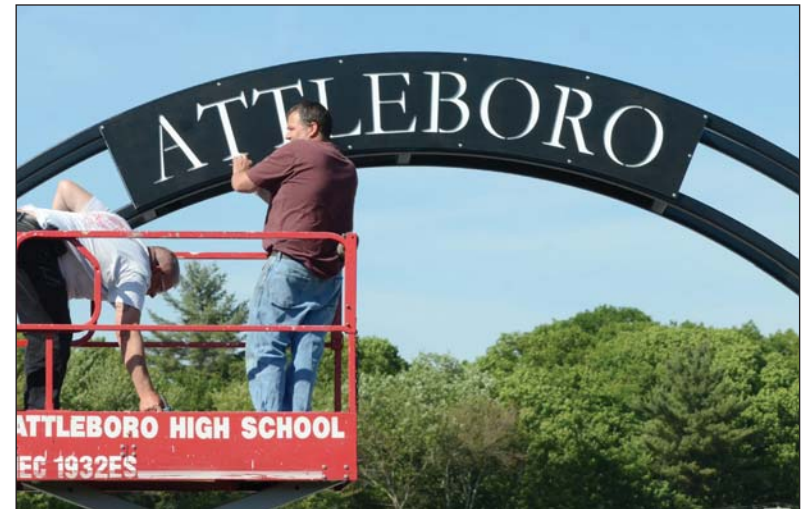
Attleboro school department employee Thomas Bodge, left, and Jeff Badger of Badger Welding, North Attleboro, work on the Attleboro sign at Tozier-Cassidy Field.
