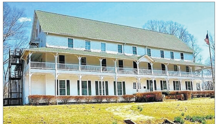
Restoration of the historic hotel at Vade Mecum is underway
