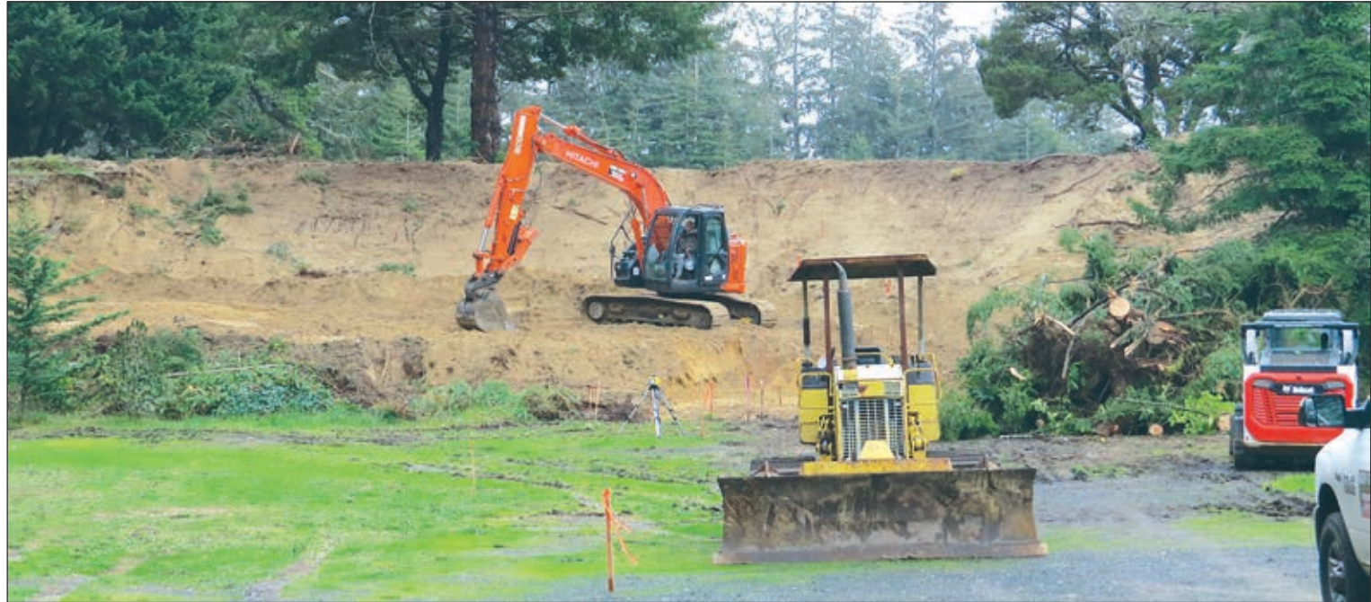
Work continues near the parking area off Highway 126. Tony Reed photos
