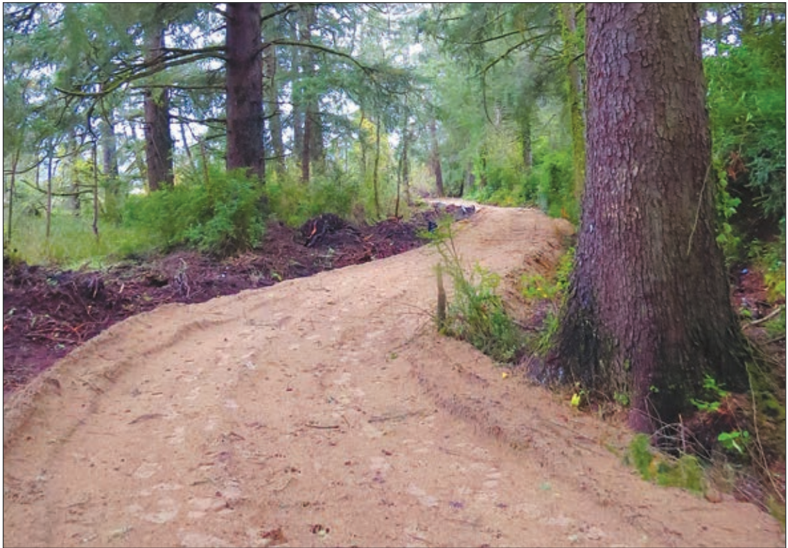
The path is in place through the trees next to the river east of the events center.
