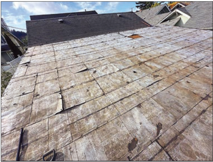
The large roof was entirely covered in old newspaper press plates before they were taken down and put to one side. Photo provided.
