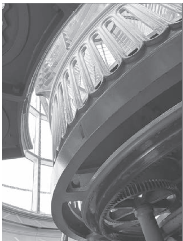
Left, the entire lens and platform inside the lighthouse is rotated by gears. Right, in the bottom right, of the photo, one of the worn carriage wheels is visible, marked with an “8.”
