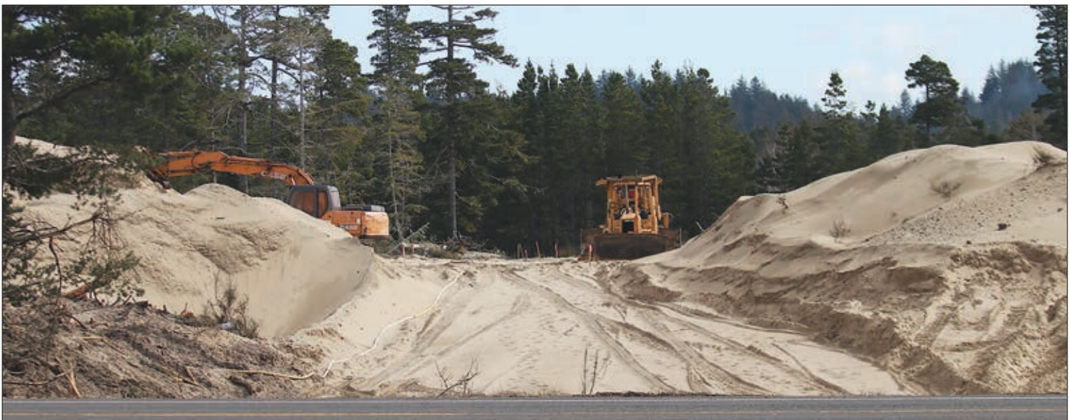
Workers and equipment are moving a lot of sand to create streets around a planned development of an assisted living facility.
