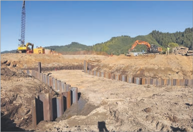
Heavy equipment seen along 126 is constructing a new channel to help stabilize salmon populations. Photo provided.
