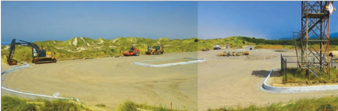
Two stitched photos show the entire parking lot at the north jetty as it waits to be repaved. Tony Reed photo.
