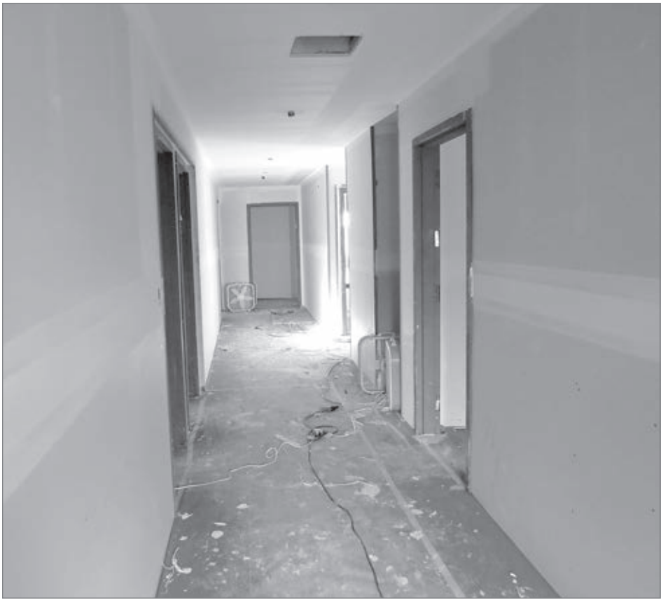
Sheet rock insulation is nearly complete on the top floor, and construction personnel are working their way down.
