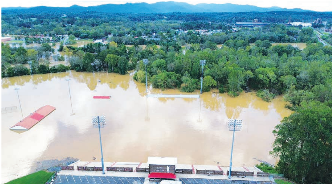
Freedom High School's football field and field house flooded as a result of Hurricane Helene aftermath.
