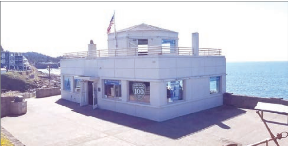
This temporary closure will allow the contractors to complete essential roof replacement work. (Courtesy photo from the OPRD)
