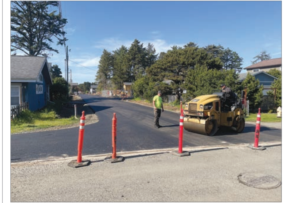
The paving of Northwest Biggs Street between Northwest 58th Street and Northwest 60th Street in north Newport was completed last week. This roadwork is related to the construction of the Samaritan Treatment and Recovery Services (STARS) adult residential and outpatient center, which is currently scheduled to be opening to patients in early September, with a public celebration being held in late August. (Photo by Steve Card)
