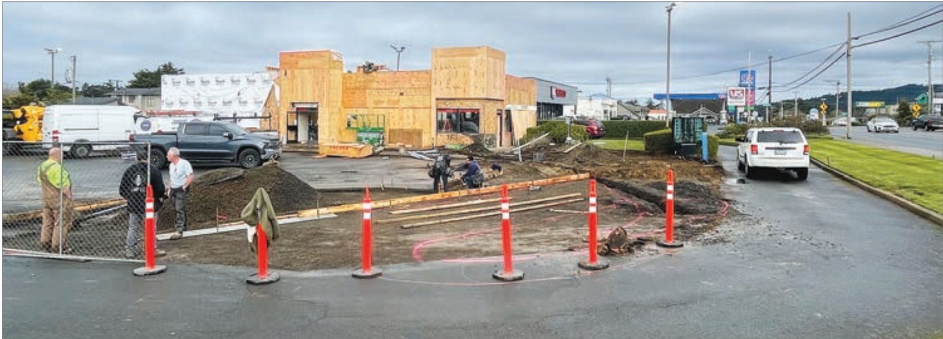
Burger King in Newport is undergoing some major reconstruction work, both inside and outside the building. The project is slated for completion by mid May. (Photos by Steve Card)
