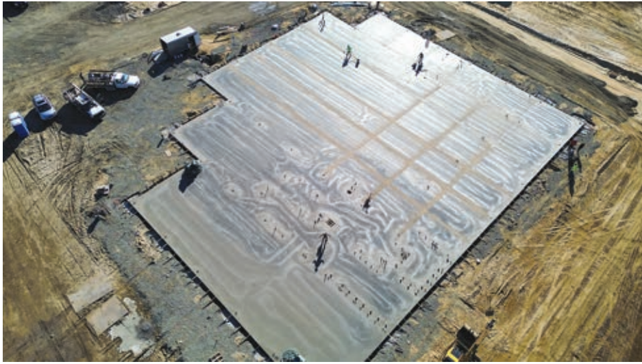
This aerial view shows the recently poured foundation for the new, 20,000-square-foot South Beach Church. The site, located at 301 SE 40 th St., includes 12 acres of land. (Courtesy photo)
