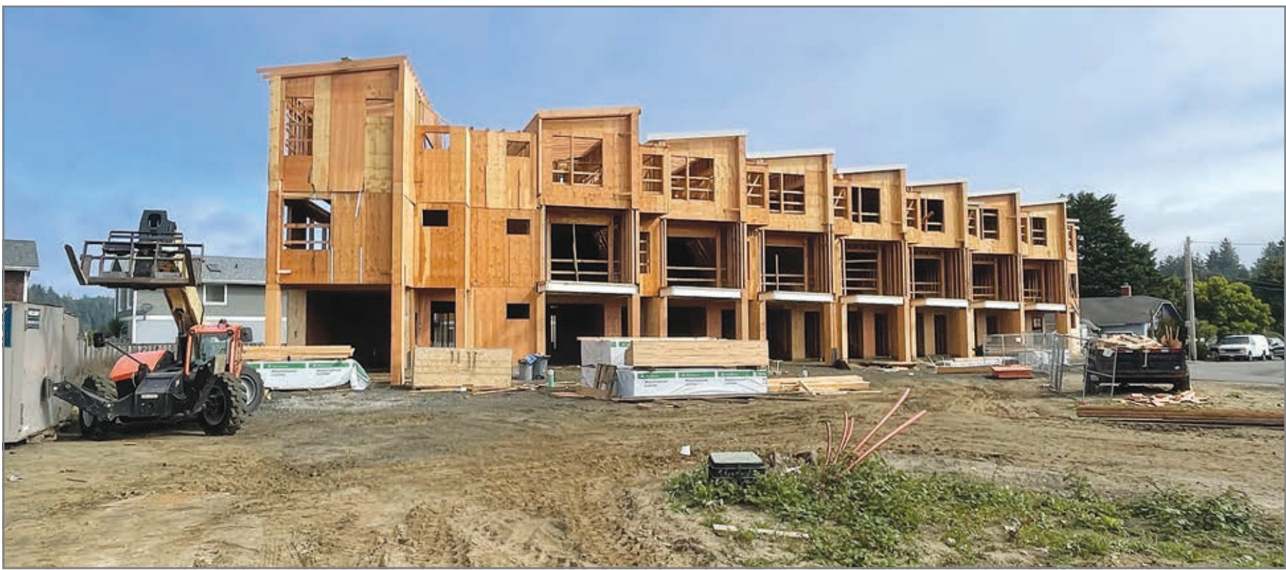
An eight-unit townhouse complex is under construction in Waldport near the intersection of Cedar and Huckleberry streets. This is located in what's known as Waldport's downtown district, which has a special zoning that allows mixed commercial/residential use. These are going to be just residential, and, according to a city official, the developer has indicated that he is going to start off using them as short-term rentals. (Photo by Steve Card)
