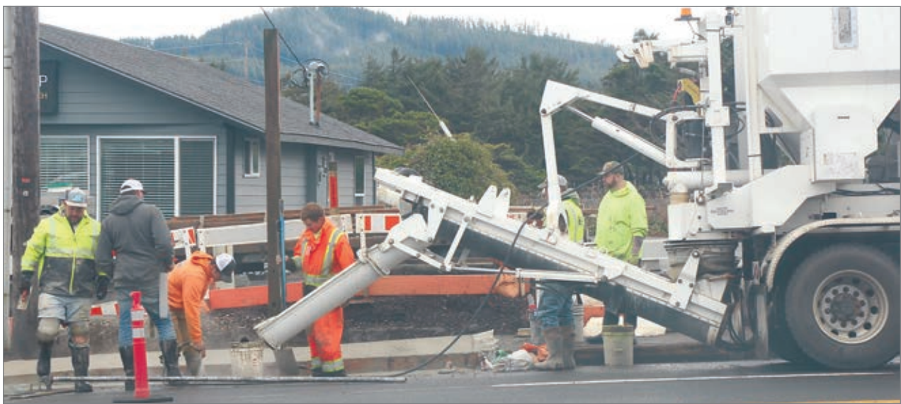
Oregon Department of Transportation crews have been upgrading the curb ramps along Highway 101 in Lincoln City. (Photo by Jeremy C. Ruark)
