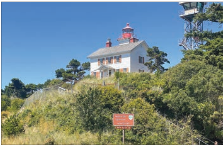
The Oregon Parks and Recreation Department is seeking bids for major renovation work on the exterior of the Yaquina Bay Lighthouse in Newport. A total of $1.4 million has been allocated for the project, which will include the repair of roof framing, chimneys, brick foundation, lantern, siding, doors, and windows with the installation of a new roof and complete exterior paint coatings. Bids for the project will be opened Aug. 15, with a deadline of June 30, 2025, for completion of the project. (Photo by Steve Card)
