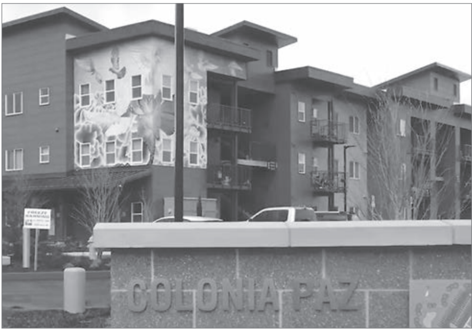
Farmworkers live in this affordable housing project in Lebanon. A new housing program will help Oregonians on Medicaid receive up to six months in rental assistance. (Courtesy of Oregon Health Authority)
