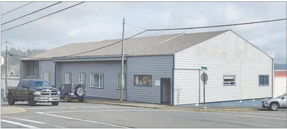
The shelter facility at Seventh and Hubert Streets in Newport is undergoing renovations, could welcome overnight guests after the new year. The First Presbyterian Church, located at 227 NE 12th Street, is the current Newport winter shelter. (File photo)
