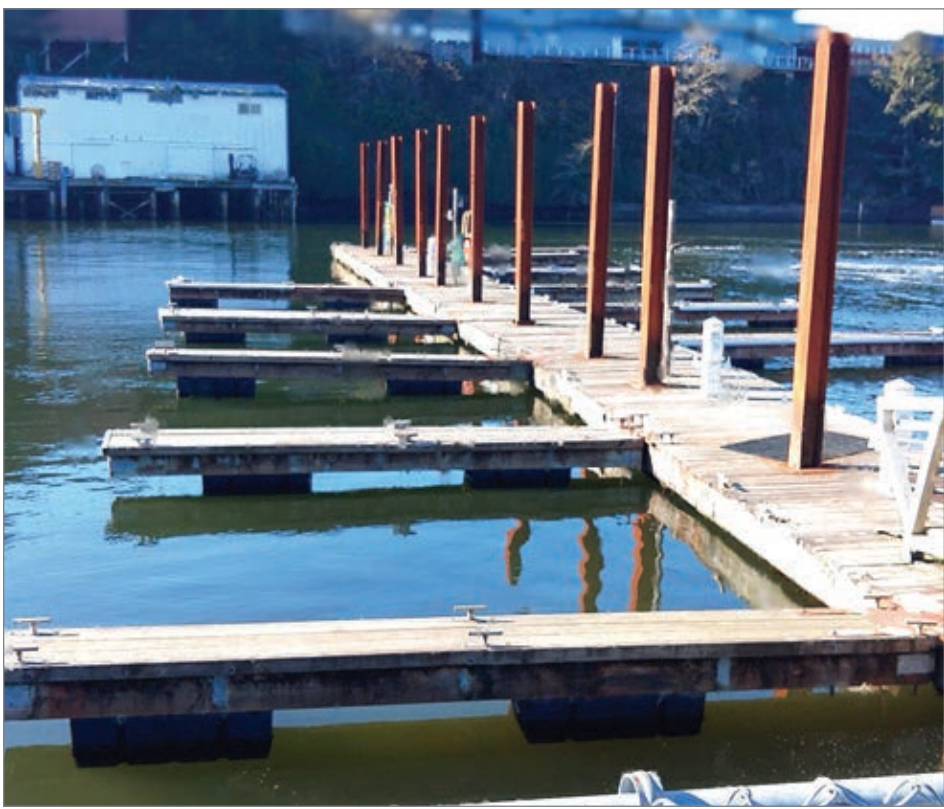
The old wooden docks at the Depoe Bay Harbor were more than 75 years old and in bad shape. They have now been replaced with four new docks. (Courtesy photo)
