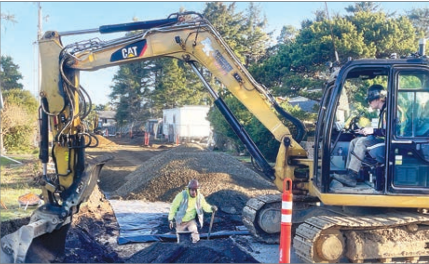
Work is continuing on improvements to Northwest Biggs Street in north Newport. A water main along the street was installed last year, and work is now underway to build up the road and prepare for paving. This road work is related to the Samaritan Treatment and Recovery Services (STARS) adult residential and outpatient center scheduled to open this summer. Work on Biggs Street is scheduled to continue into May, with traffic at times being reduced to one lane. (Photo by Steve Card)
