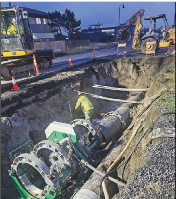
Repairs have been completed to Newport’s treated effluent pipeline in South Beach. The effluent wastewater, which is treated, chlorinated water, was being diverted into Yaquina Bay since late December. (Courtesy photo)
