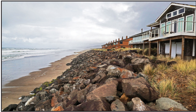
Oceanfront landowners in Neskowin have chosen to use rock revetments, or rip-rap, to protect their properties from erosion.
