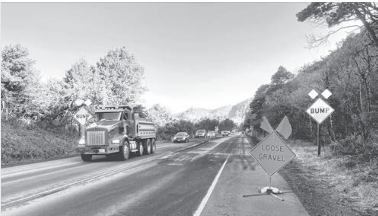
One lane of Highway 101 near Beverly Beach State Park was closed last week while work was underway to once again smooth out that section of roadway. (Photo by Steve Card)
