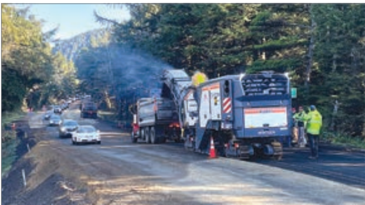
Road crews were busy last week grinding up damaged asphalt and laying new pavement along a stretch of Highway 101 at Beverly Beach. (Photo by Steve Card)
