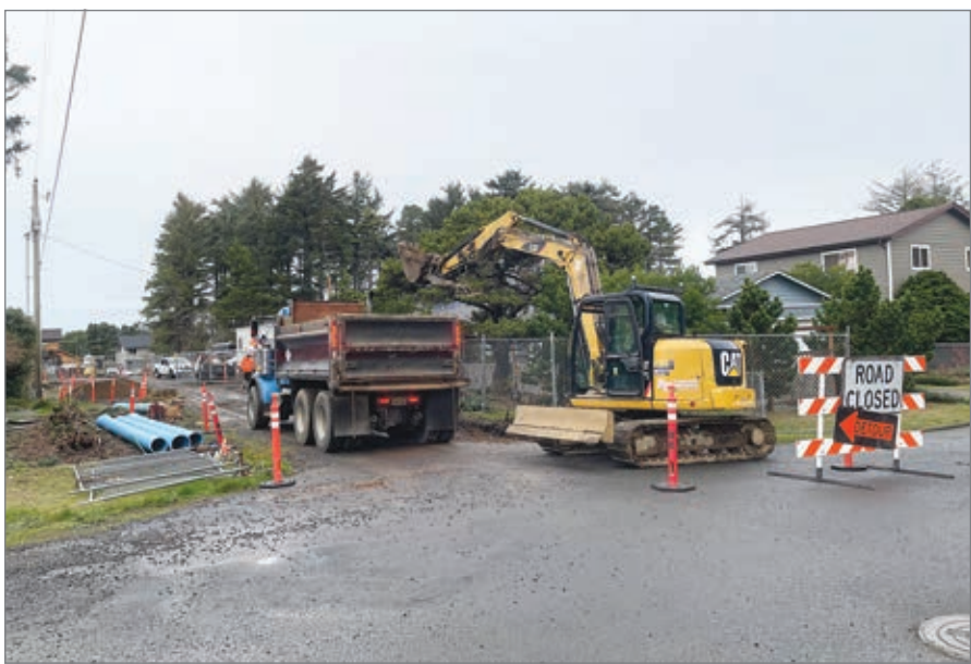
A new water main was installed last week along Northwest Biggs Street in north Newport. The project was necessary in order to supply water to the future Samaritan Treatment and Recovery Services (STARS) adult residential and outpatient center currently under construction there. (Photo by Steve Card)
