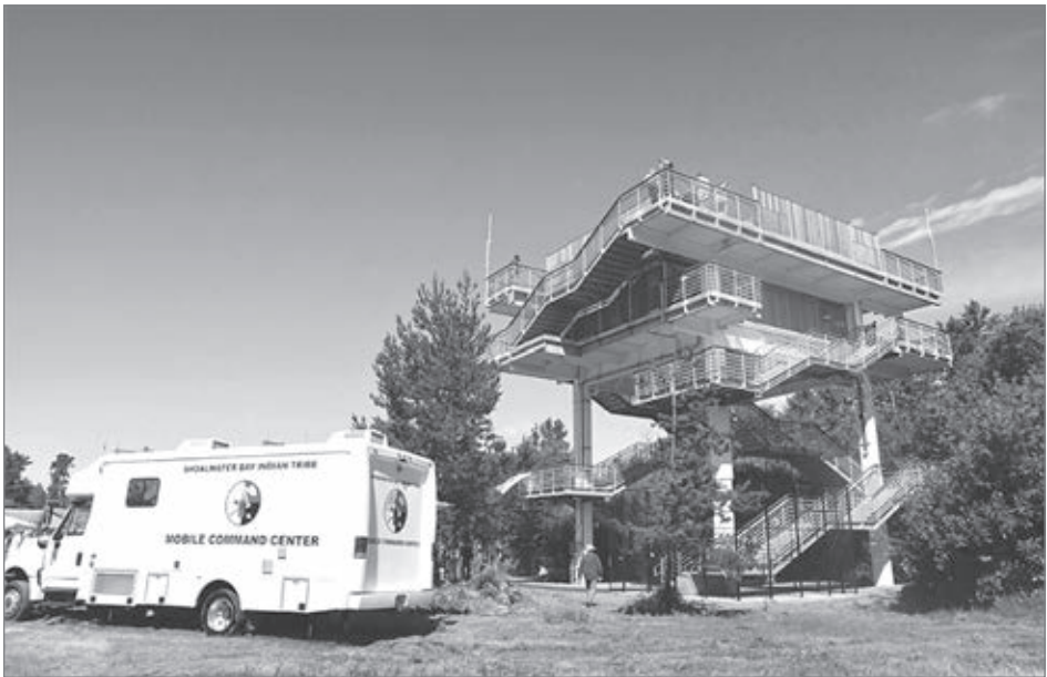
Shoalwater Bay Tribe Tsunami Tower - Tokeland, Washington. (Courtesy from the Washington Military Department)
