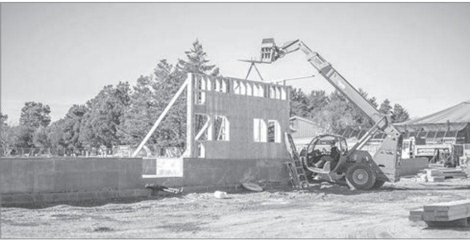
During construction last March, the walls were put into place for the Oregon Coast Aquarium’s new marine wildlife rehabilitation center. (Courtesy photo from Jeremy Burke)
