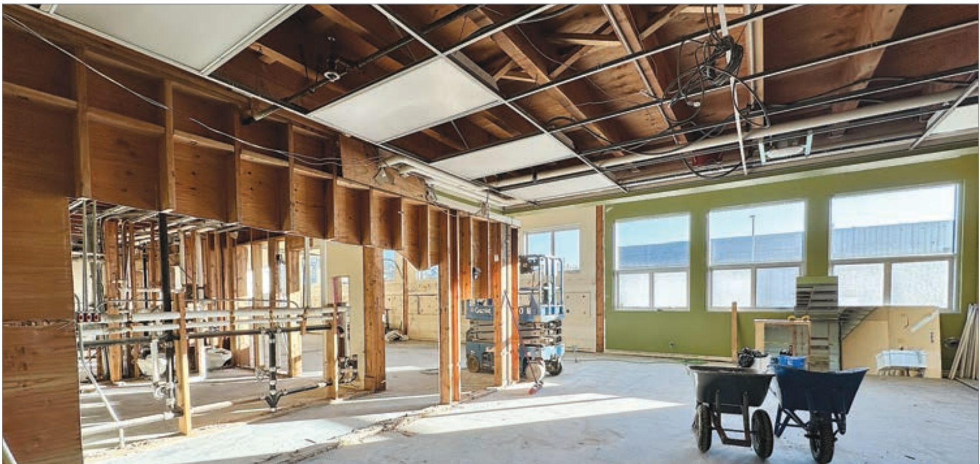
The final phase of the Capital Campaign to renovate the Newport Performing Arts Center is nearing completion. The public is invited to help outfit new backstage spaces — and even add their own names to this beloved community building. (Courtesy photos)
