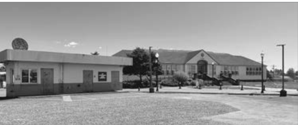
This building next to Newport City Hall used to house a gas station. The structure will be demolished and the property redeveloped. (Photo by Steve Card)
