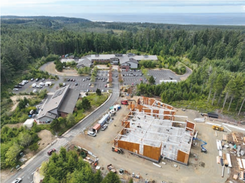
On May 21, 2024, voters in Lincoln County approved a bond measure referred by OCCC to build a center for trades education and update and upgrade existing college facilities. This flyover shows work at the Newport campus. (Courtesy photo)
