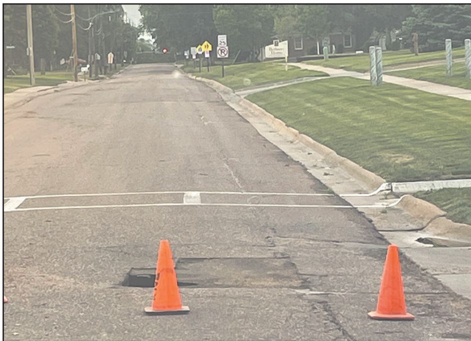
A corroded culvert recently collapsed resulting in sinkholes on 1st Street near the intersection with Blaine Avenue. The street will be closed for repairs for approximately two weeks. (Courier photo by Chance Eikenberry)
