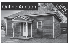
405 McKelvey St. - Bladen 2 Bed, 1 Bath, storage shed
