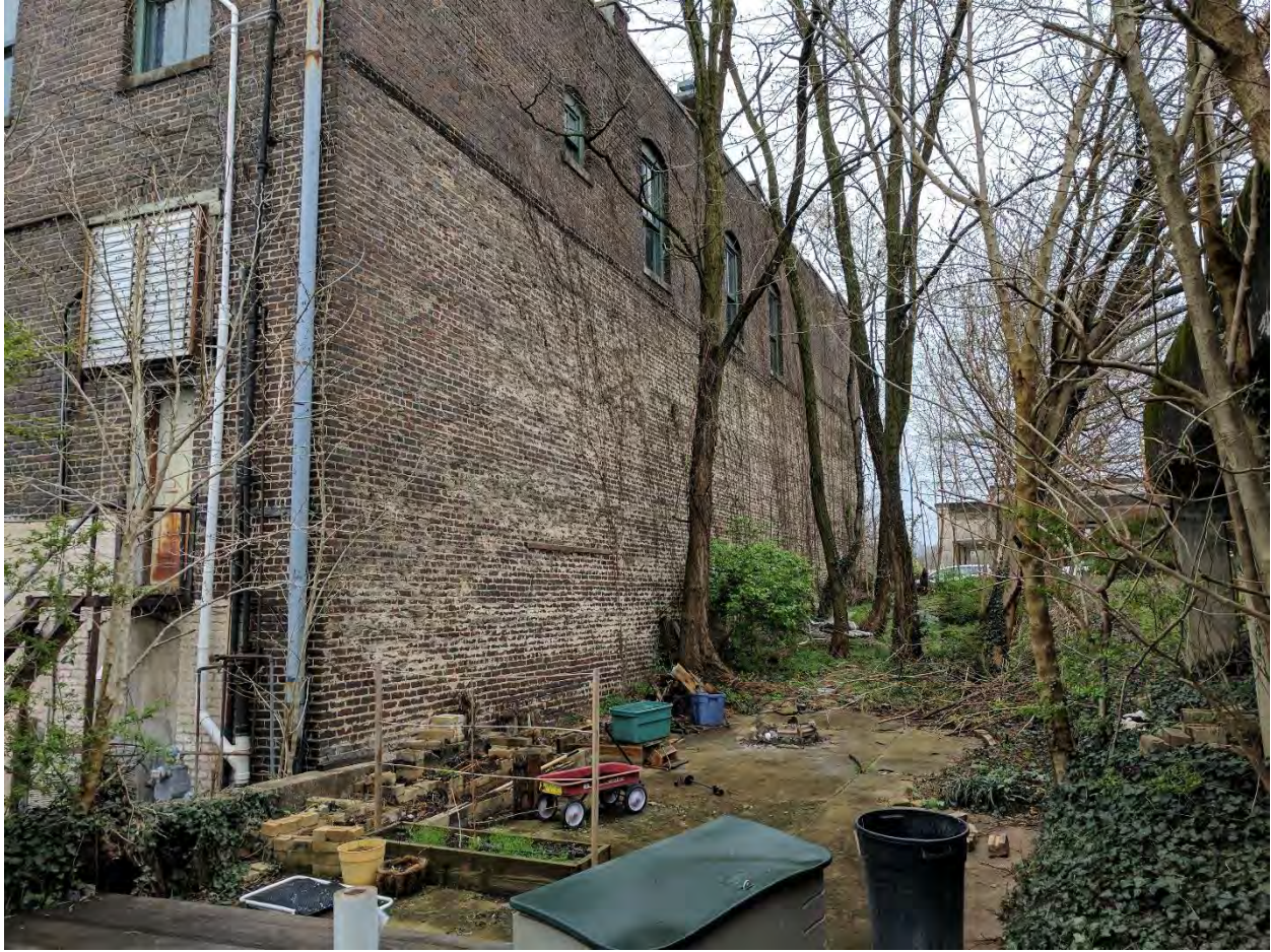
View of facade facing the vacant lot
