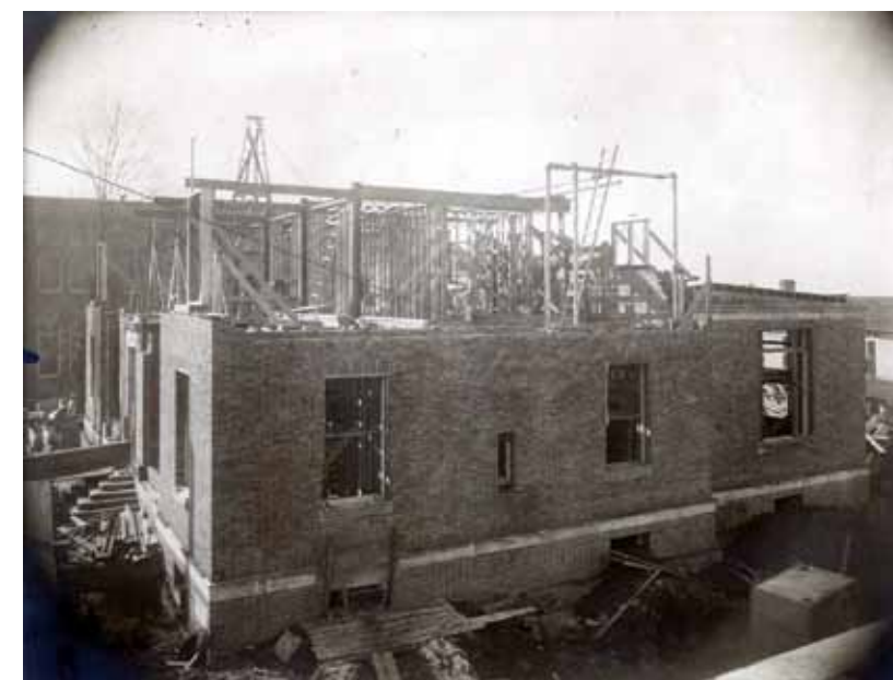
Federal Post Office framing – December 1916
