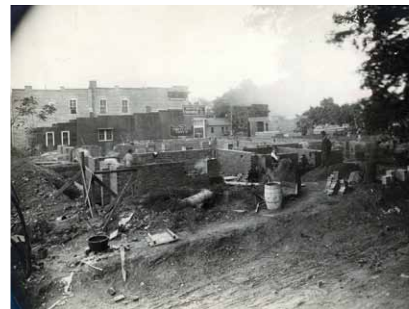
Federal Post Office foundation – October 2, 1916
