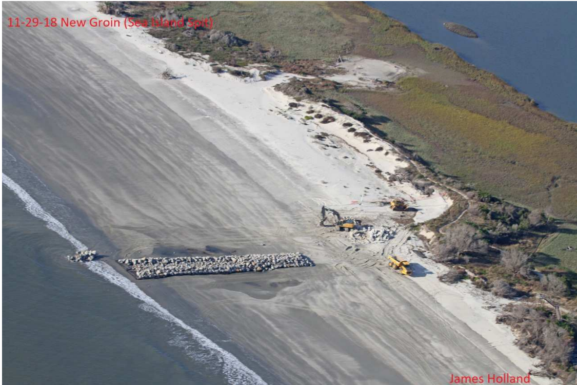
Photograph taken November 29, 2018 by James Holland showing ongoing construction
