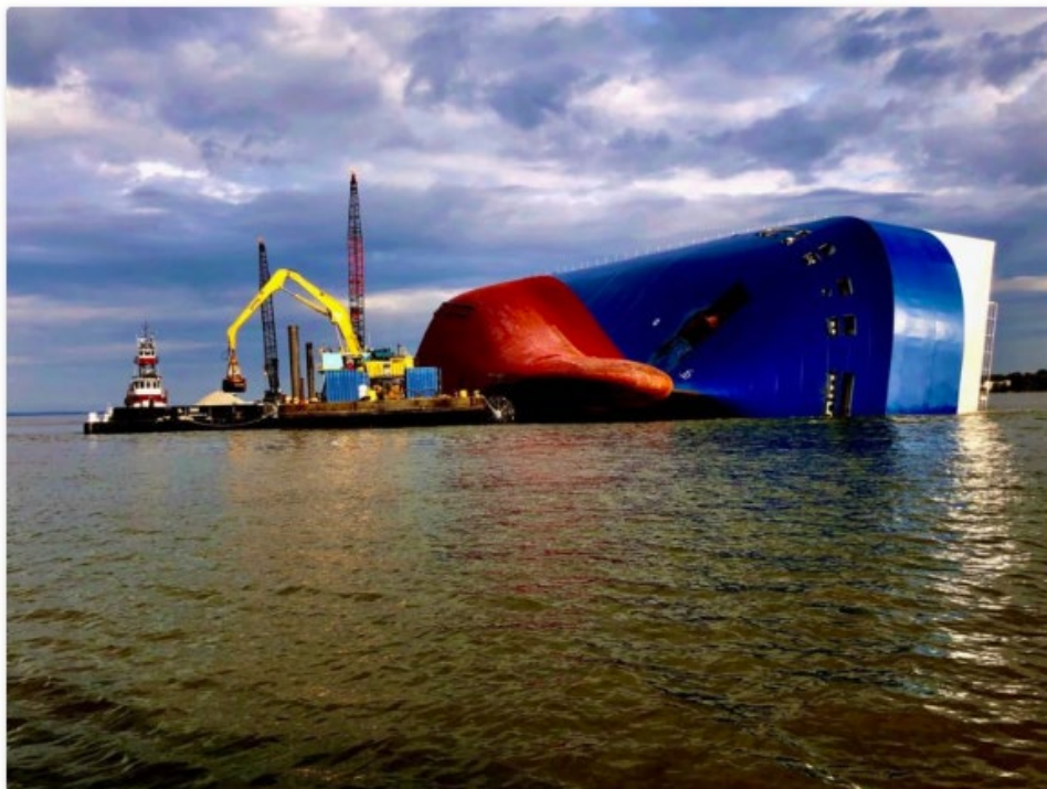
Donjon-SMIT laying down rocks to stabilize the GOLDEN RAY
