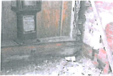
Corner at storefront pilaster
