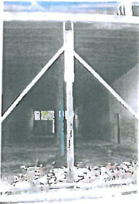
Column at Grant Street
