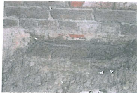
Exposed brick ledger/wall footing
