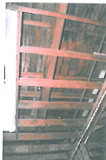
Bottom cord of ladder truss on ceiling joists
