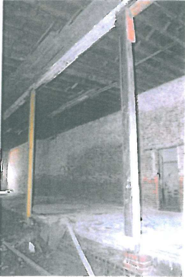
Temporary columns under old beam
