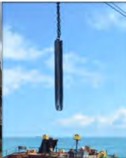
Figure 14 Chisel operated by a free fall crane.
