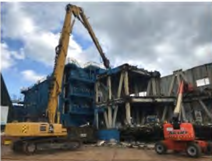
Figure 15 Long Reach excavator with shears used in demolition ashore.
