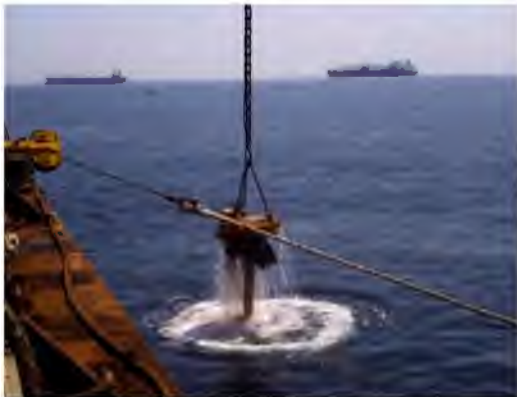
Figure 10 An electromagnet being used during a sub-surface debris removal operation
