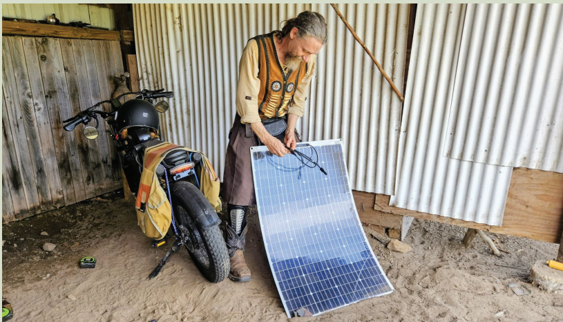
Joe Guthrie works at building out a charging station in a lean-to for his electric bike.
