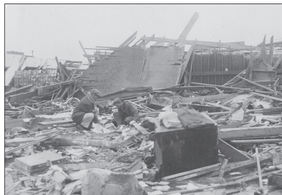
Indiana State Library Archives/National Weather Service Homes in the McCaw subdivision demolished in Princeton, Indiana.
