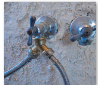
Modern laundry detergents work fine in cold water. Turn off the hot water supply to your washer and reduce your water carbon footprint significantly. With a wye supplying cold water to both the hot and cold inlets, the washer will not stall if someone selects hot water.
