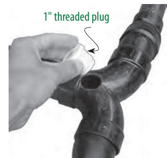
A flow-splitter retrofitted with inspection access. The access is sealed with a threaded plug.
