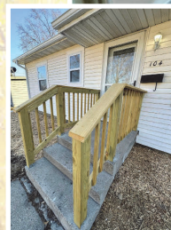
Exterior repair or upkeep
