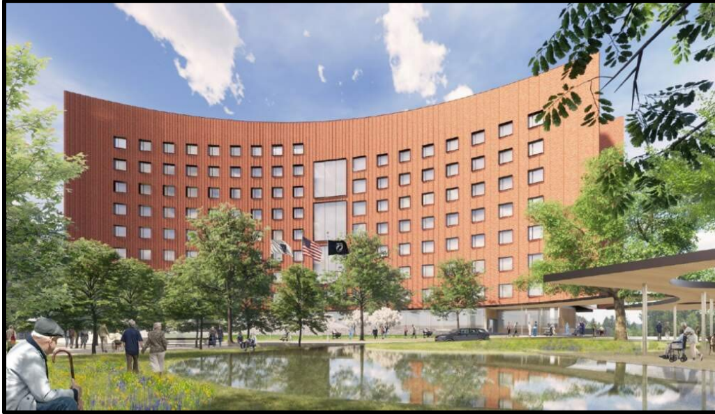
Figure 4 :The new Veterans Home in Holyoke's long-term care facility, scheduled to open Fall 2028
