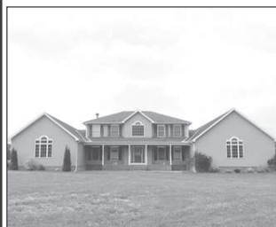
Plymouth Twp $699,000 Large 4 BR/ 2.5 BA Colonial Home on 84 acres. Attached Garage & detached Garage & barn. 2 gas wells & pond. #4014869 Lois Blank 440-265-0820
