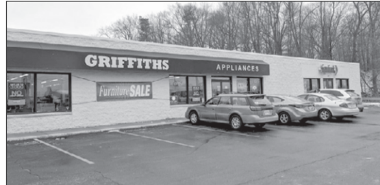
Ashtabula $699,900 Commercial building. 2 retail store fronts. Right on Rt 20. #4064413 Tom Bush 440-265-9262
