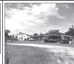
Conneaut $19,900 Commercial building at a great price! 34x56 pole building with 20x40 lean-to. #4025553 Lois Blank 440-265-0820
