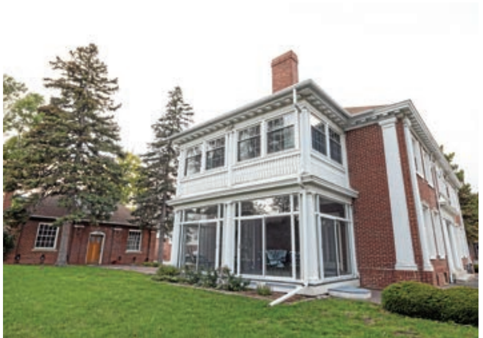
A sunroom outside the library and enclosed balcony on the second floor connected to the master wing is shown.
