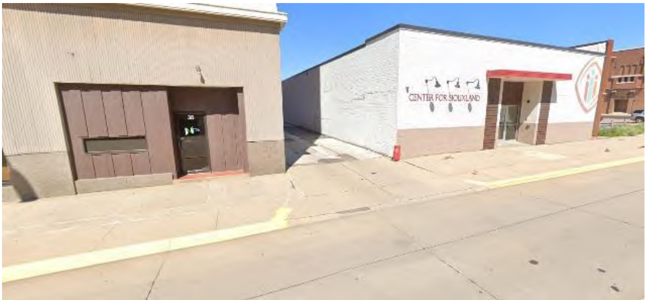
View Looking West from Douglas Street
